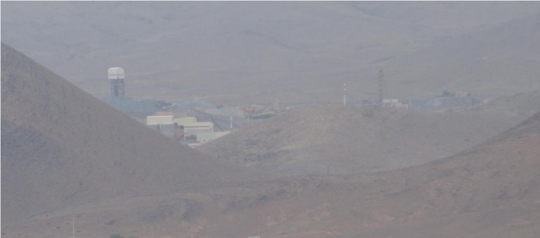
Installations of the silver mine operated by the SMI, 3 km from Imider
