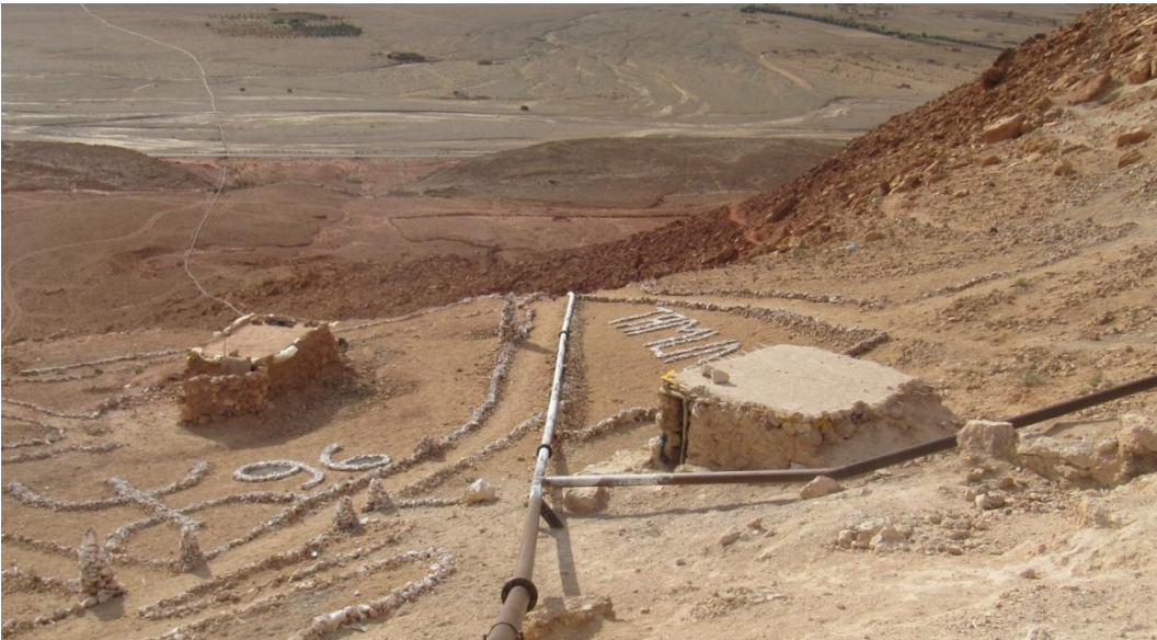
pipes bringing water to the mine
