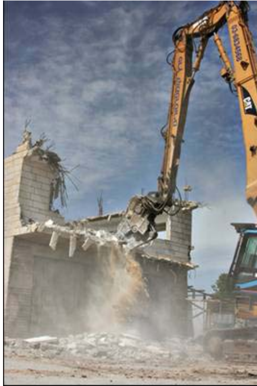
Demolition of family home in East Jerusalem (photo credit: ICAHD)
