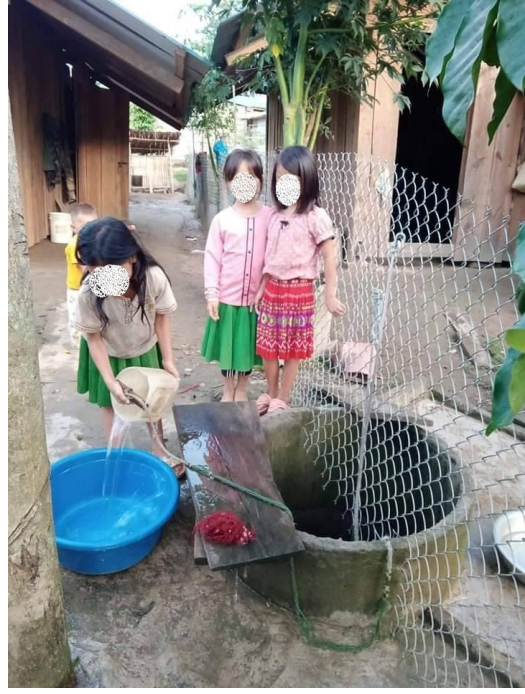
The well without proper physical safeguards
