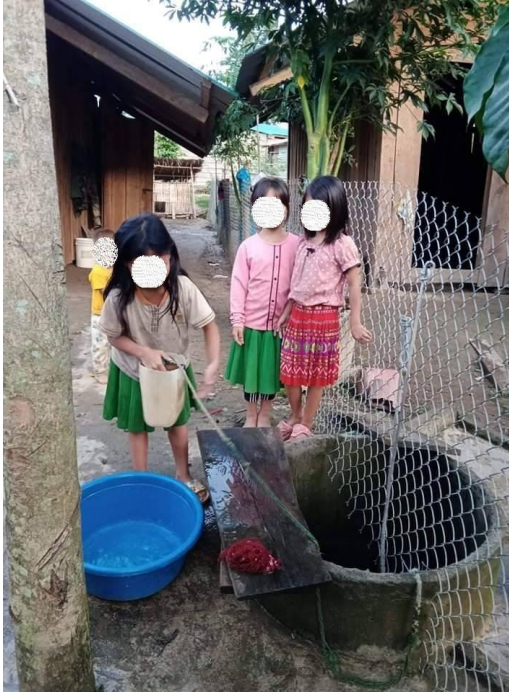
The well without proper physical safeguards
