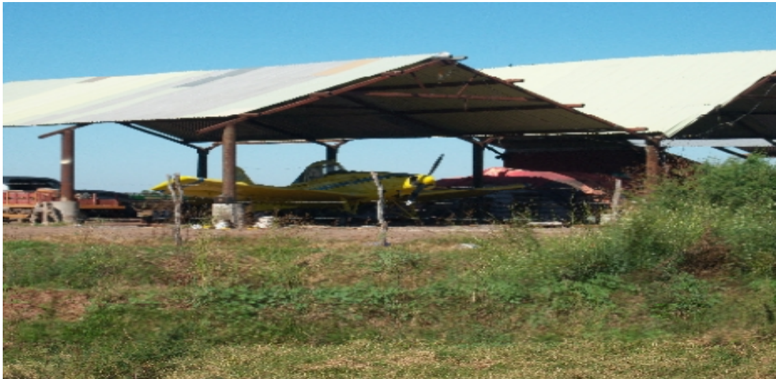
(Landing strip and plane for aerial fumigation)
