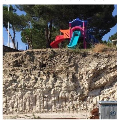
Figure 4. Photo from a playground in Gördes, Manisa, where a construction site is situated next to the playground and no safety measures are in place
